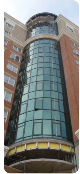
Figure 4: Curved Glass Facade
